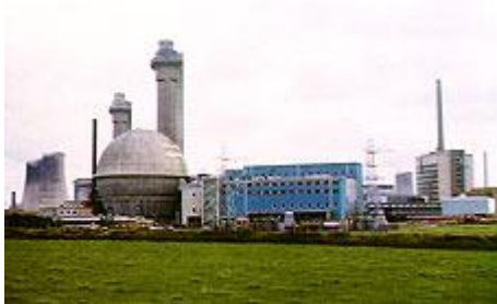
Calder Hall nuclear power station
